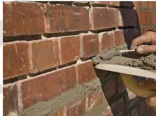
Repoint mortar joints where there is evidence of deterioration.
