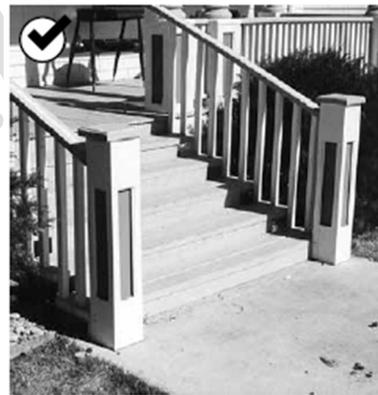
*After: Post and handrail are appropriately reconstructed.*
