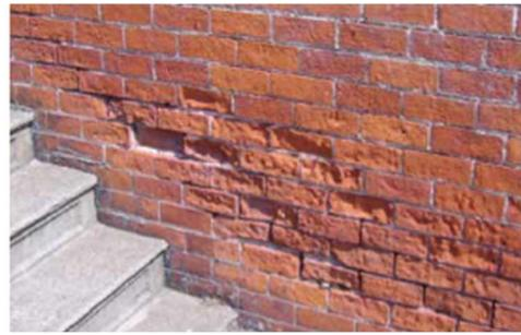
*Brick showing damage from inappropriate cleaning (photo courtesy of Heritage Ohio).*
