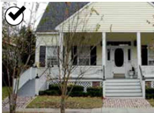
*Avoid altering character-defining features when adding a ramp. For example, this ramp is set to the side, which maintains the character of the front steps.*
